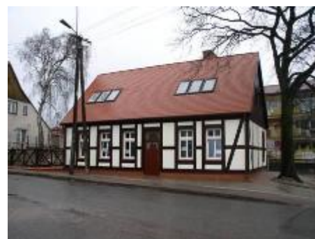
13, Kosynierów Street after rehabilitation
