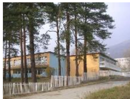
nursery school "Purvi Juni" after rehabilitation
